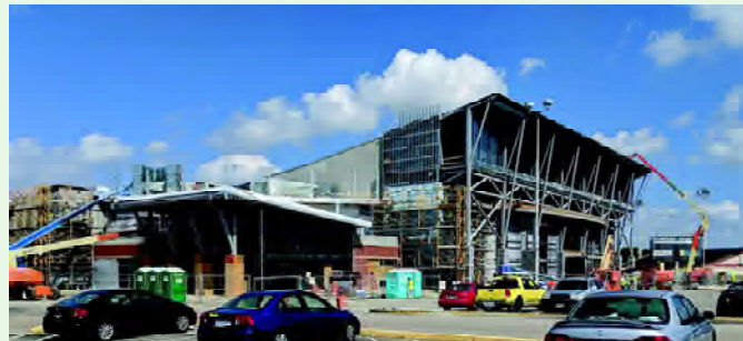
UD Arena renovation by Wagner Industrial Electric.
