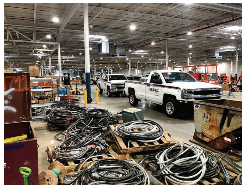
Ongoing work at Phoenix-Dayton Group.
