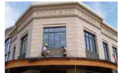
The Greene under construction
