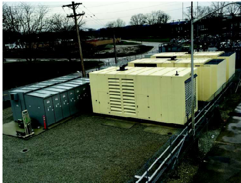
New 2 megawatt generator at WPAFB.
