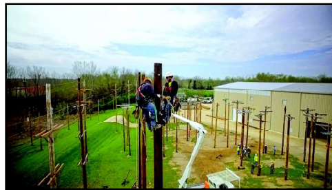
ALBAT simulates a transmission system for training on high-voltage systems including an 80-foot steel lattice tower and wooden pole structures.
